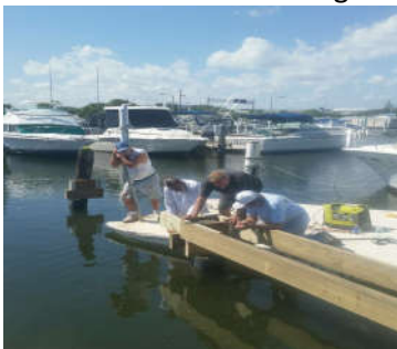
ACME Dock Rebuilding
